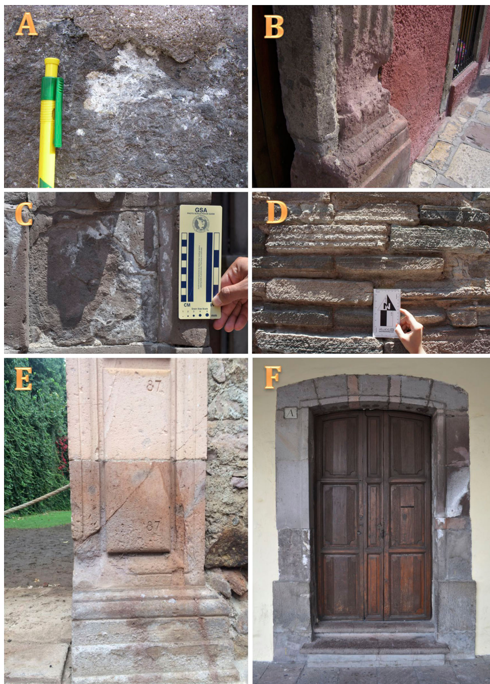
Plate 1 Different aspects of deterioration caused by salt bursting. a , b Lost material in the SG black and RG red of San Miguel de Allende. c Flaking in the ESC Tuff of Querétaro. d Sanding off in the LS Tuff
